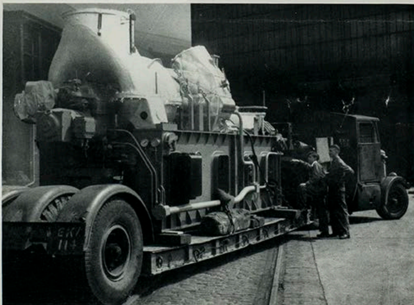
Fig. 12. Part of the gas turbine set arriving at the shipbuilding yard of R. & W. Hawthorn Leslie & Co., Ltd., Newcastle-on-Tyne, for installation on the Anglo-Saxon Petroleum Company's Tanker "Auris."
